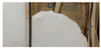
Applegate R-Foam flows across the fiberglass to slow down the flow of air. This photo shows Applegate R-Foam being installed in a wall cavity with a fiberglass batt.
